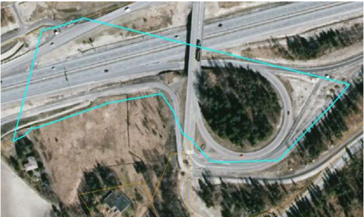
A complex intersection with a possible shift and confusion with 12220.
